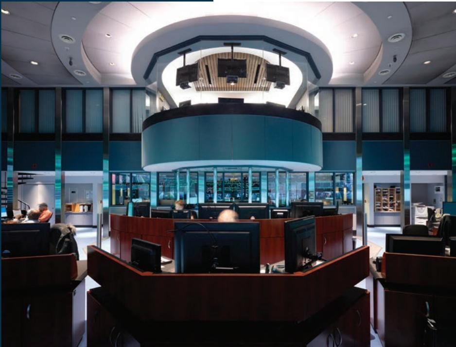
The entire project had to fit into the same footprint as the existing room, including the videowall. Sixty 70-inch video cubes are configured in three horizontal rows of 20 displays each, arrayed in a 9° arc, left to right.
